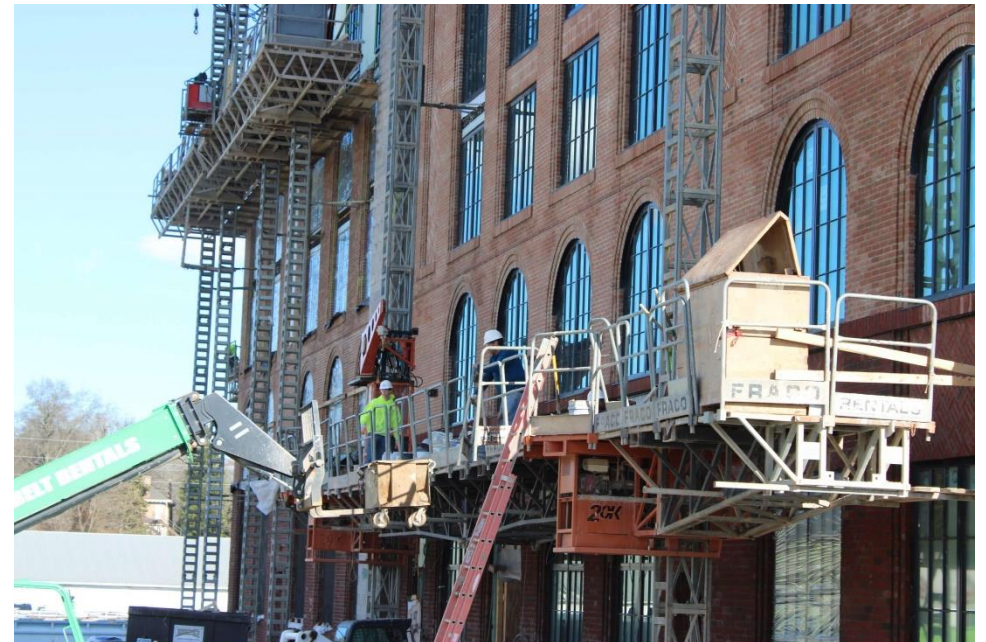
TDA Project: The Manchester Hotel
